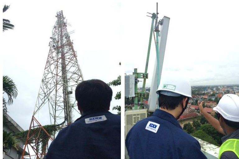
Taken in Yangon (2015/7/23) MPT and KSGM (KDDI Summit Global Myanmar Co., Ltd.) staff involved in base station facility expansion
